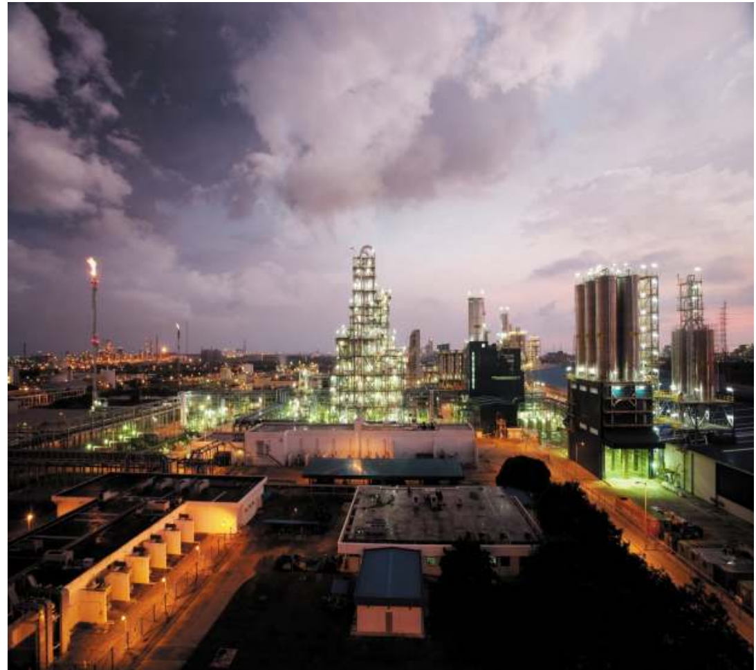
<Thailand, HMC PP Project >
